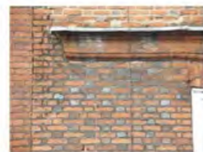
Red Brick with burnt headers: Flemish bond
